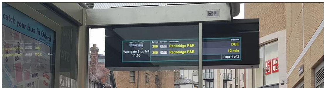
Figure 2 TFT display that is mounted behind a half end glass panel. © M2M Tech
